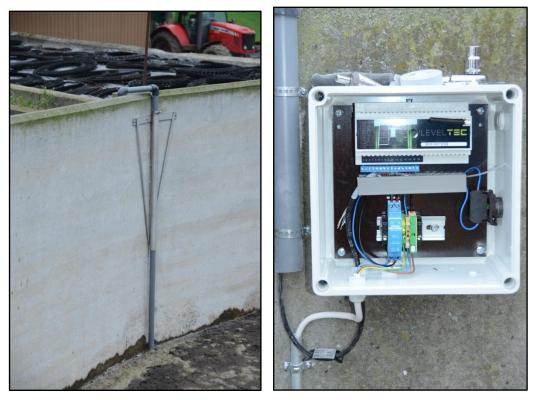
Figure 4. The photo on the left shows the PVC tube installed on the inner side of the tank wall. The photo on the right shows the control unit installed on the outside of the tank wall.
