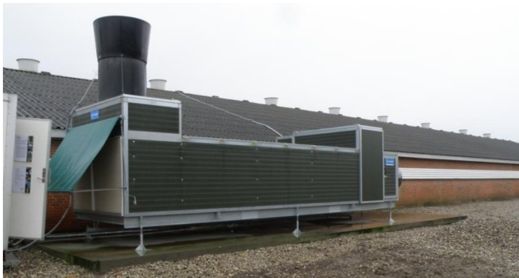
Figure 3. Picture of the Agro Clima Unit situated outside a poultry house. Ventilation air to and from the poultry house are drawn through the Agro Clima Unit by a counter current principle to utilise the heat content of out flowing air to heat up inflowing air.
