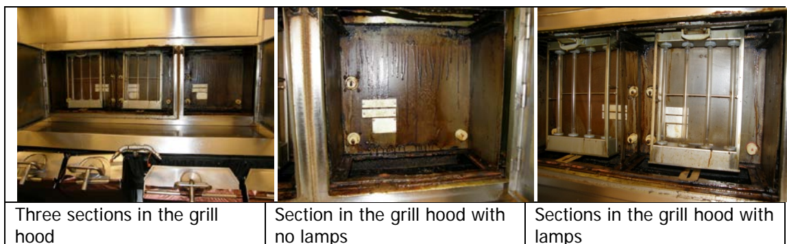
Figure 6 The interior of the grill hood with the JIMCO KPC system switched on – after 53 days
