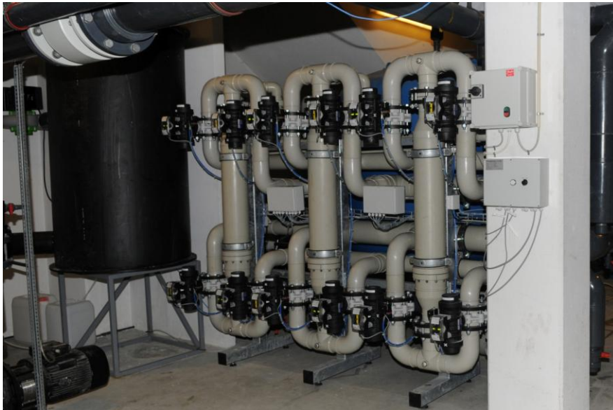
Figure 1 Provital filtration plant tested in Gladsaxe Svømmehal.
